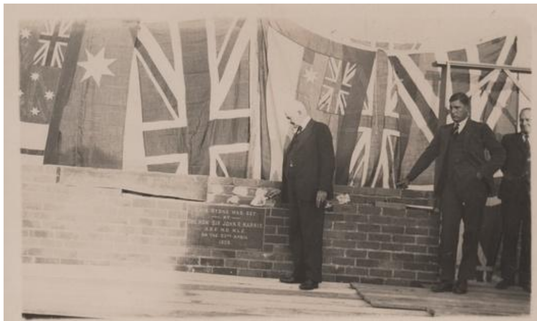
Black and white photograph of the laying of the Foundation Stone by Sir John Harris MLC for the Rutherglen Bush Nursing Hospital on 23rd April 1938.
